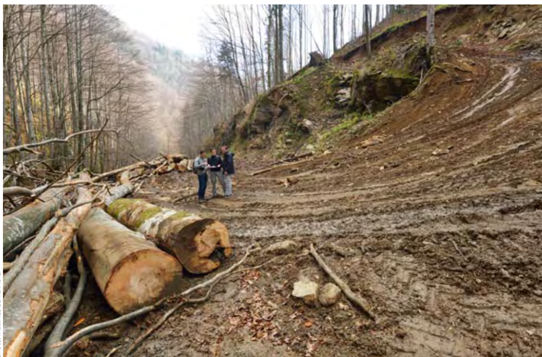
Bulldozing of logging road through the buffer zone of a UNESCO World Heritage site within Domogled - Valea Cernei National Park.
